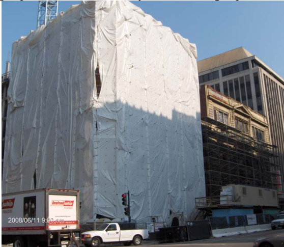
Fig. 2 – B&W Building Façade Restoration
