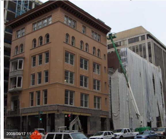
Fig. 3 – Corcoran Building Façade Restoration
